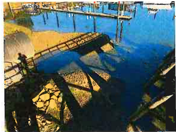
Photo 7. Sediment Impacts to Travel Lift
