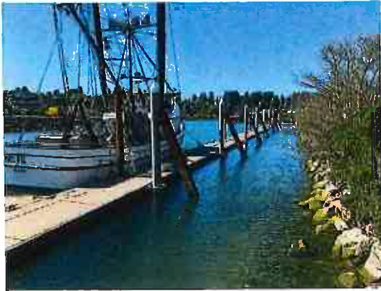
Photo 2. New Transient Dock Piling
