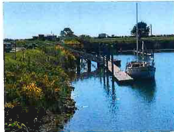
Photo 3. New Work Dock Piling
