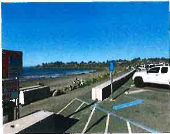
Photo 6. New Block Seawall
