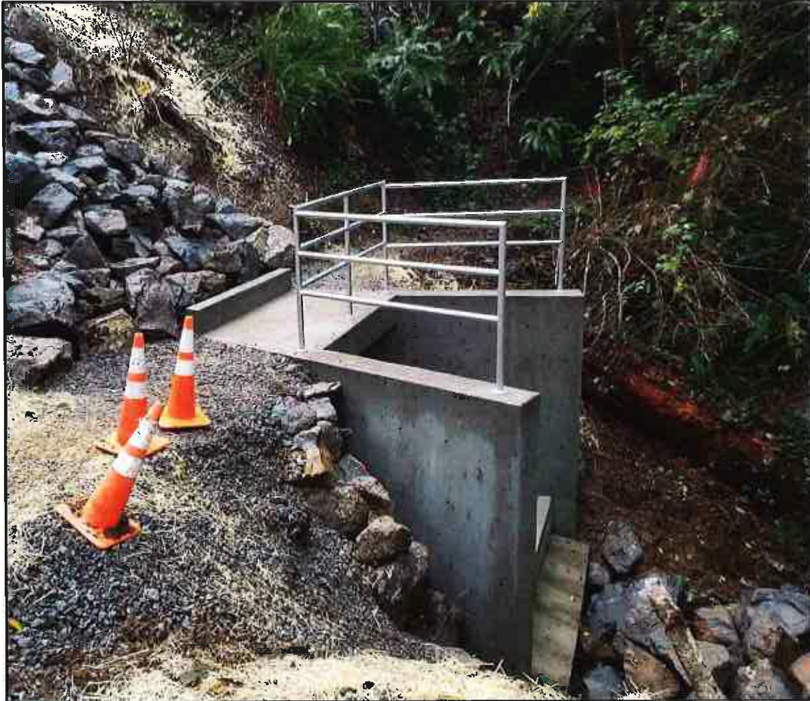
FIGURE 5.2.1 CULVERT ENDWALL STRUCTURE
