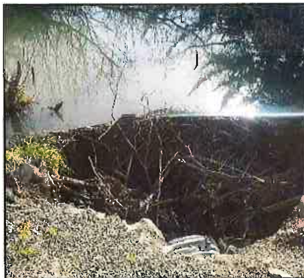
FIGURE 3.3.7 BEAVER DAM – OLD COAST ROAD MP 0.784
