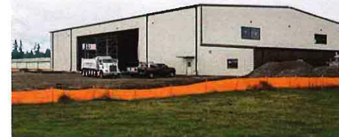
A 31,500-sq-ft building is under construction for new tenant Titan Aviation.
