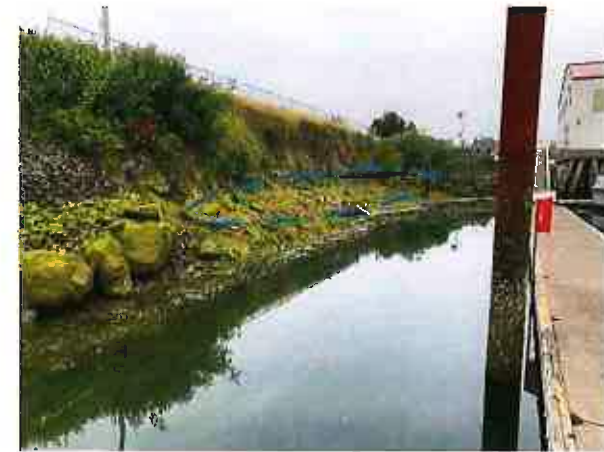
Above heavier rock intact here, but scouring is undermining embankment.
