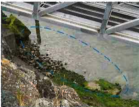
Above heavier rock intact here, but scouring is undermining embankment.
