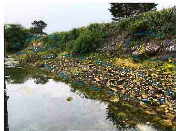
Overtopping, rutting, unraveling of rock structure. Photos show smaller rock apron, but above, heavier rock covered.
