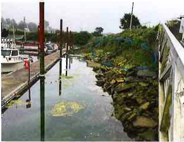
Embankment Slides and pore erosion, rock covered and/or unraveled.
