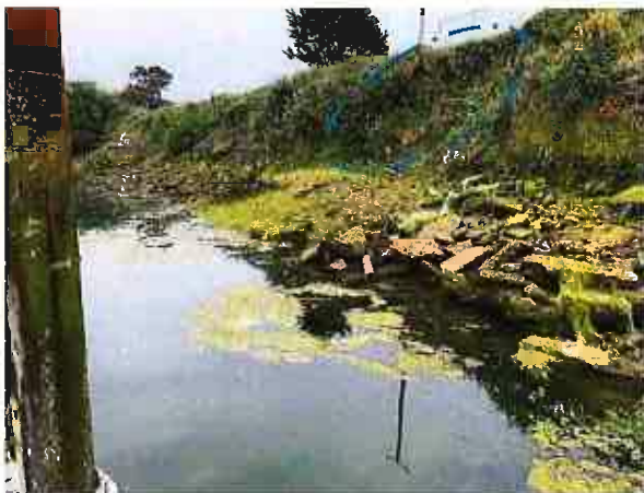
Overtopping, rutting, unraveling of rock structure. Photos show smaller rock apron, but above, heavier rock covered.
