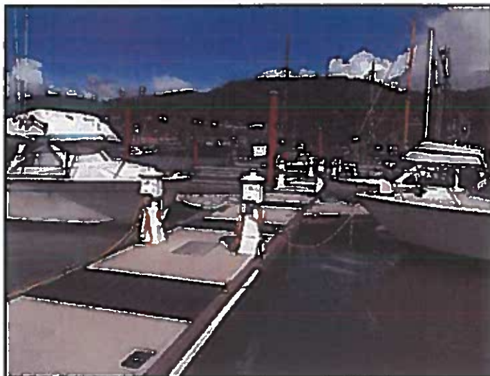
Photo 14 - New docks at commercial basin
