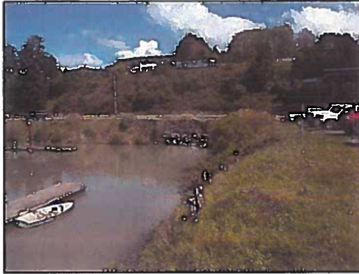
Photo 19 – Southeast corner embankment
