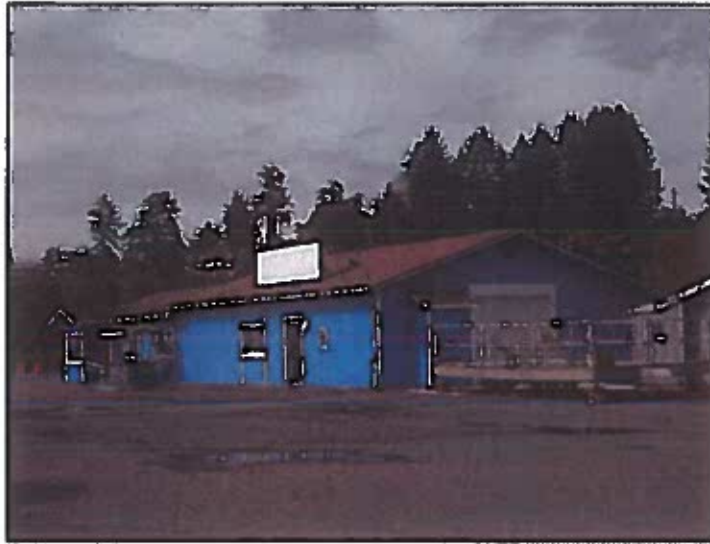
Photo 29 - Former cannery building
