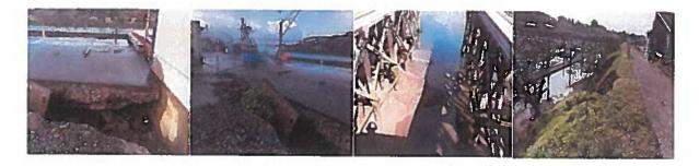
The second phase would repair 100-foot section of broken, unusable commercial receiving dock for Pacific Seafood. The reconstruction of this broken section of receiving dock would increase productivity and therefore creating twenty (20) to twentyfive (25) family wage jobs along with continued support to the local economy. Other Port infrastructure repairs would include dredging vital areas of the harbor, basin slope failures, dilapidated sewer facilities, etc.
