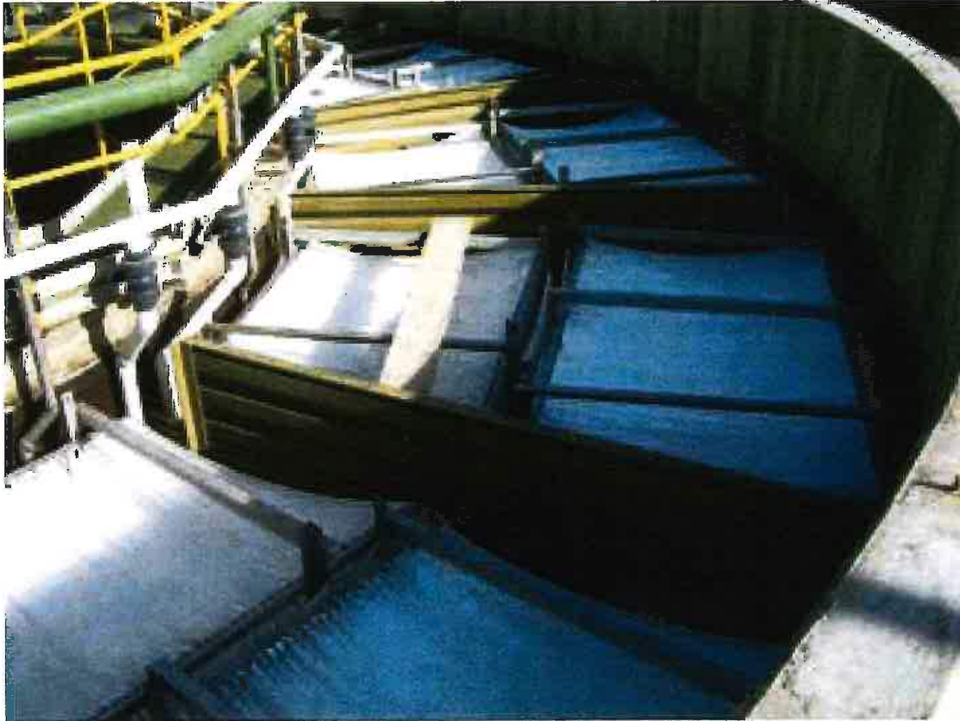
Treatment Stages with Fixed Biofilm Media
