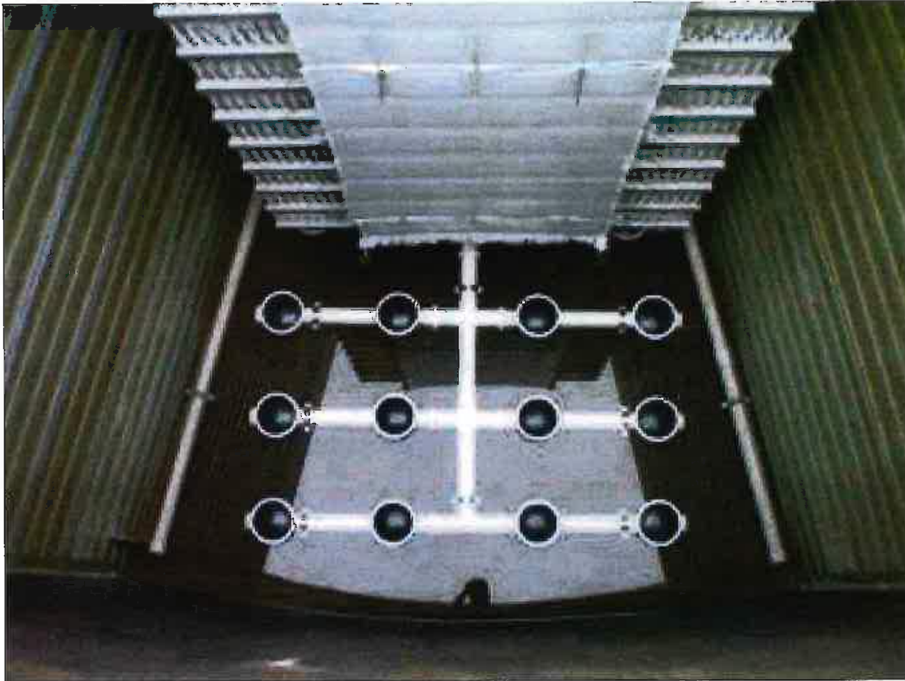
Aquarius Fine Bubble Diffused Aeration Provides High Oxygen Transfer Efficiency (OTE) and Media Scouring
