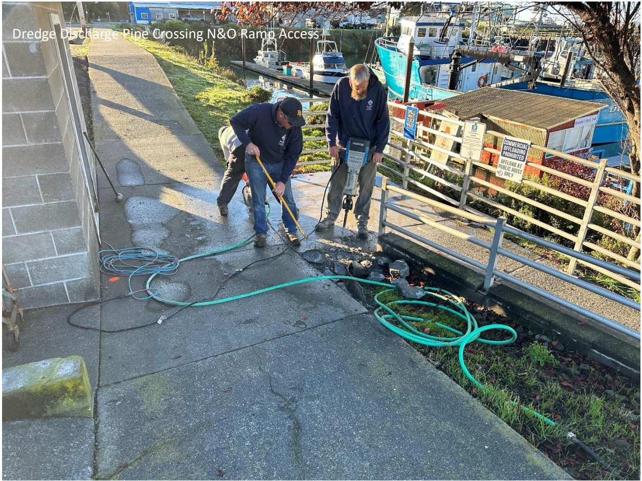
Dredge Discharge Pipe Crossing N&O Ramp Access
