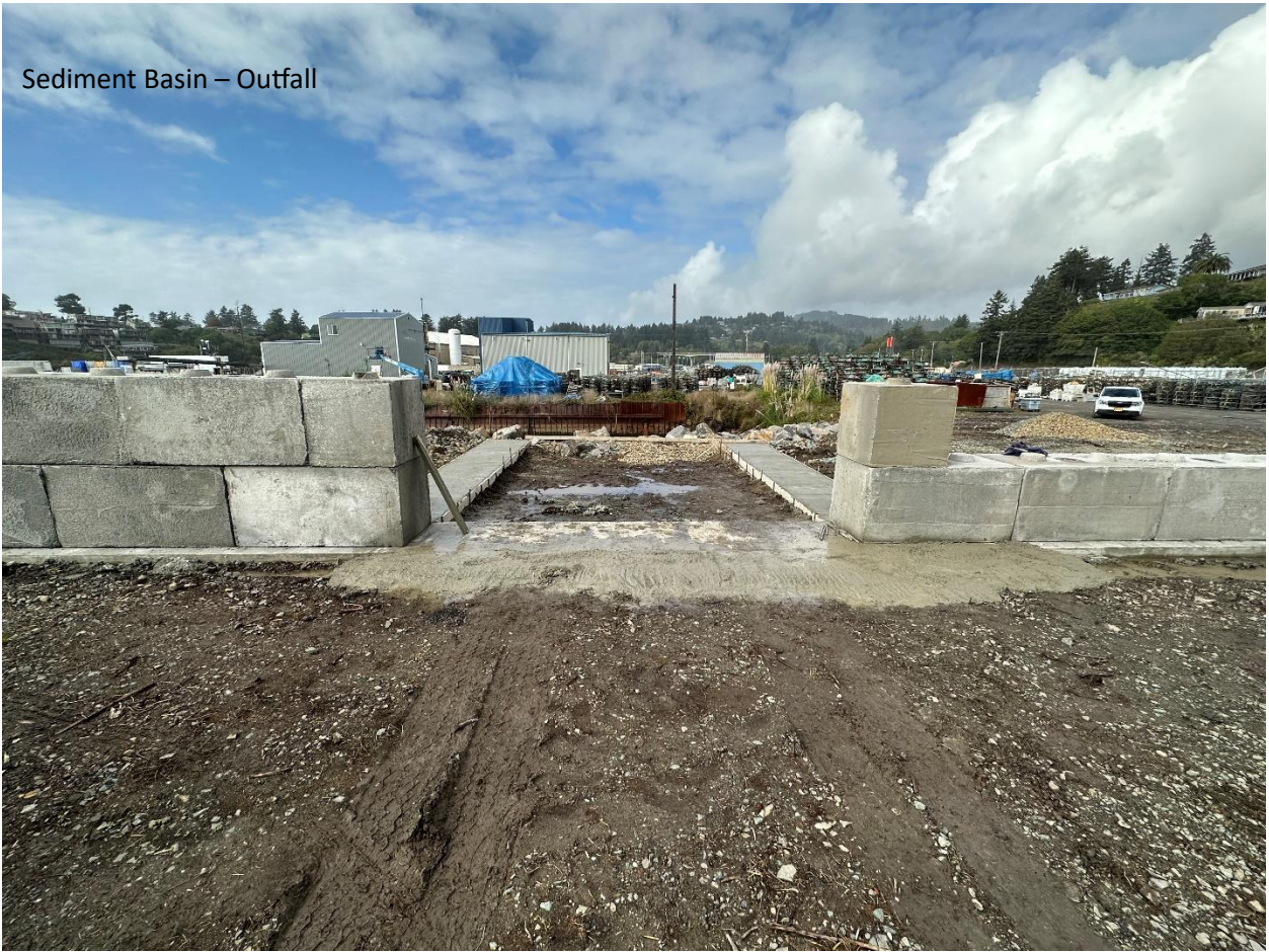
Sediment Basin – Outfall
