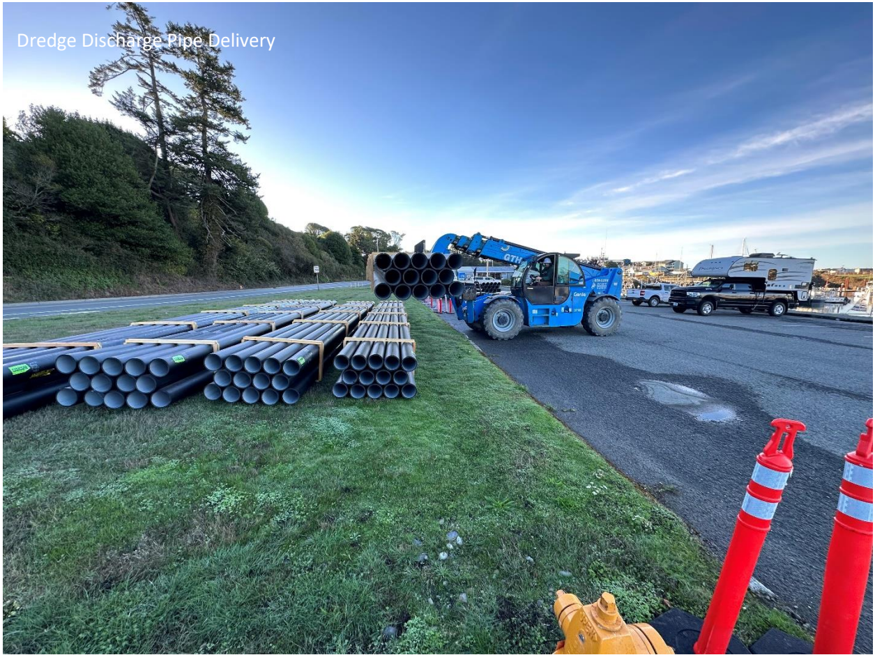
Dredge Discharge Pipe Delivery
