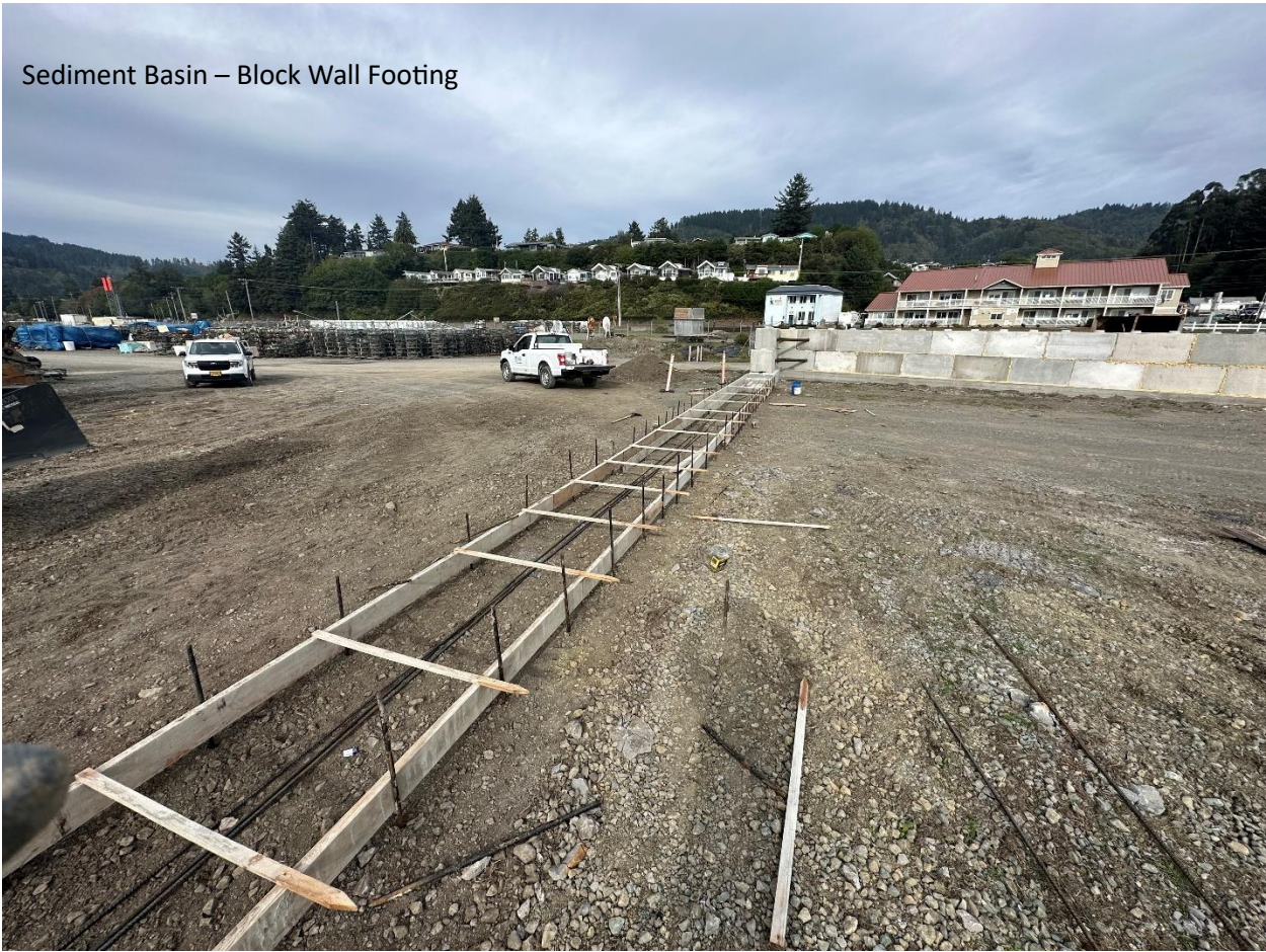
Sediment Basin – Block Wall Footing
