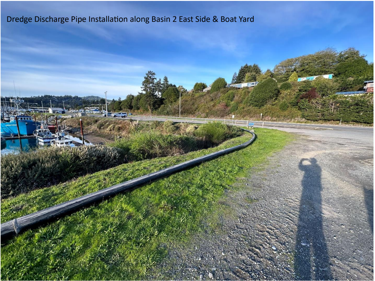
Dredge Discharge Pipe Installation along Boat Yard
