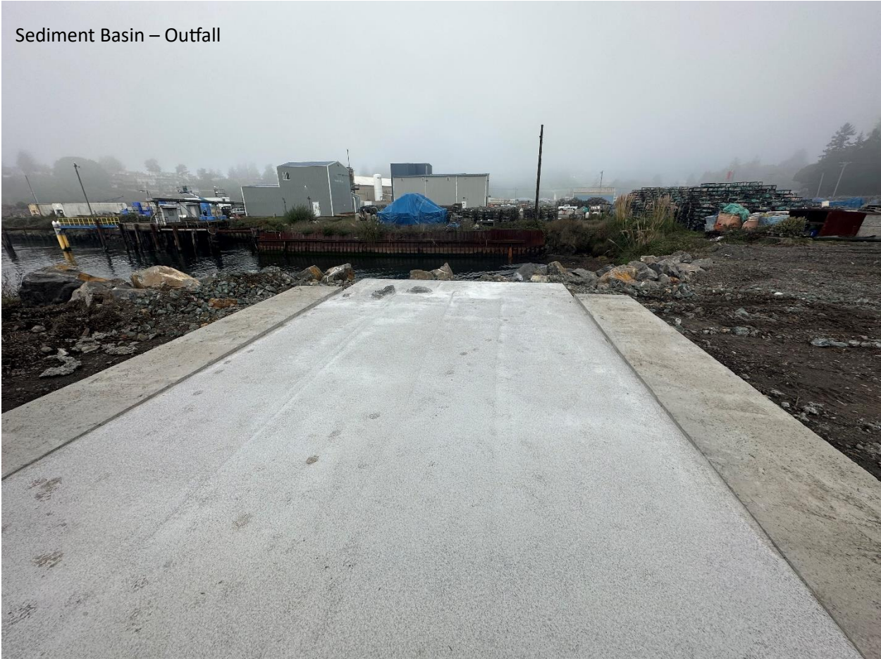
Sediment Basin – Outfall
