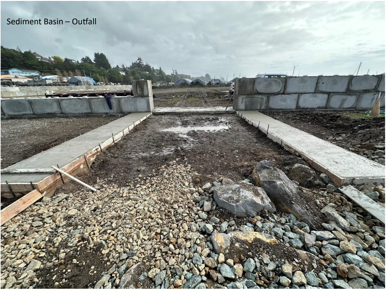
Sediment Basin – Outfall
