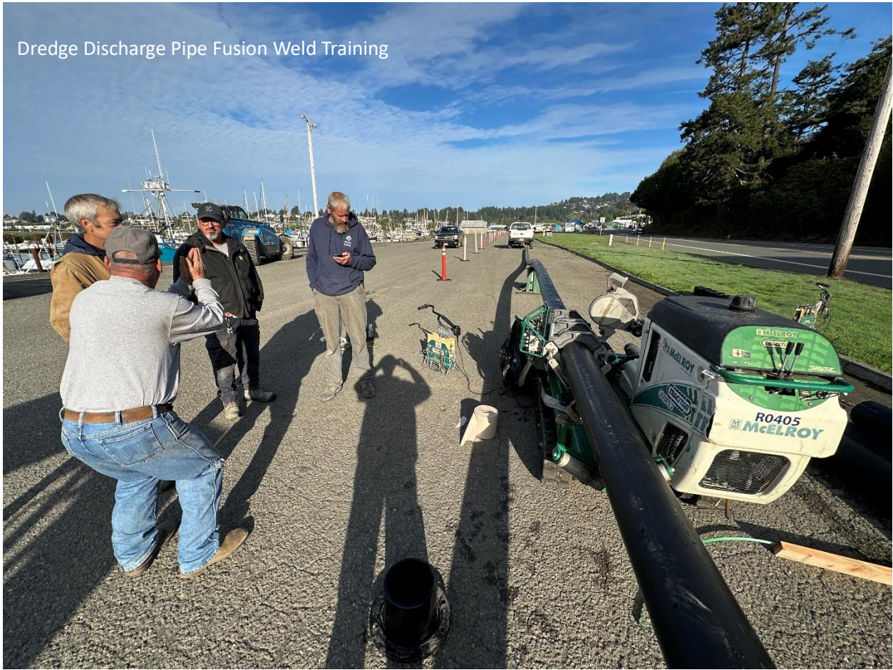
Dredge Discharge Pipe Fusion Welding
