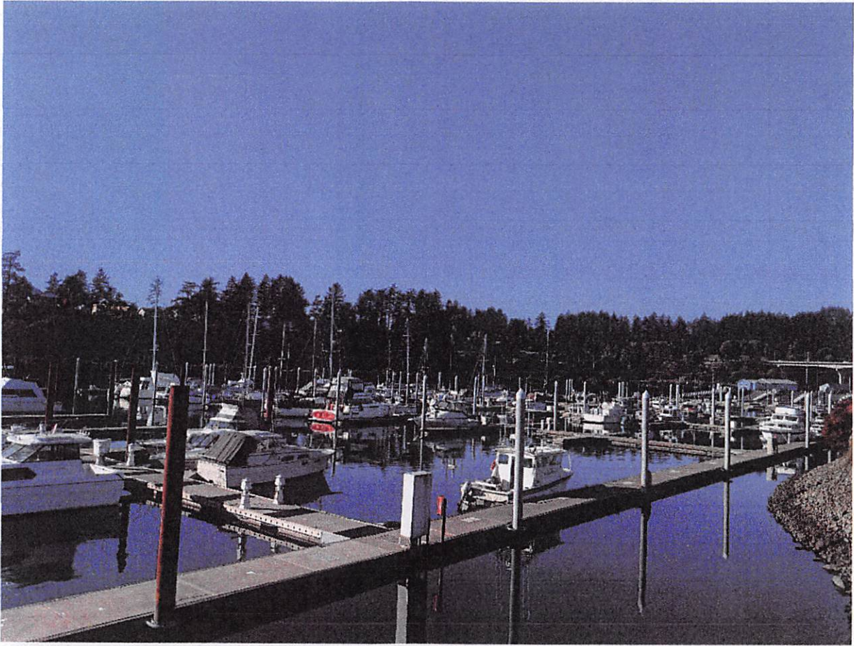
FEMA DR-4258 Basin 1 Piling Project completed April 2019
