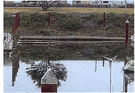
Photo 1. Closed Basin 2 C Dock
