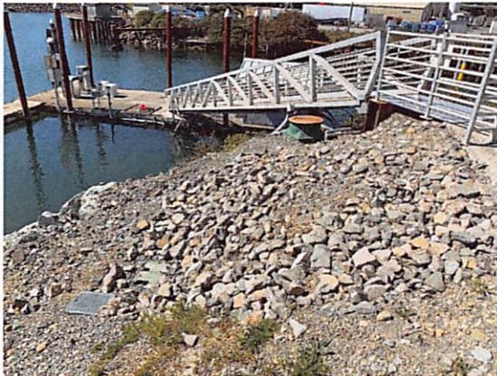
Photo 4. New Fuel Dock Ramp
