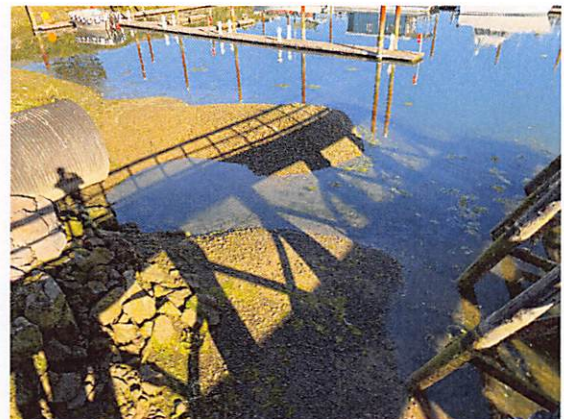
Photo 7. Sediment Impacts to Travel Lift
