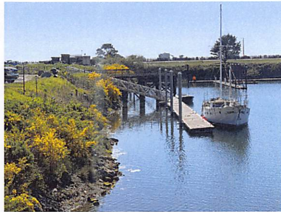
Photo 3. New Work Dock Piling
