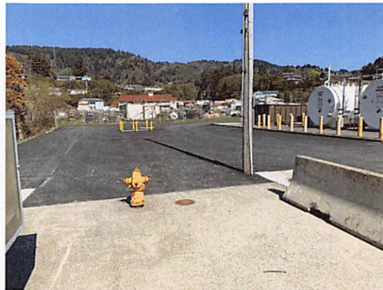
Photo 5. New Restoration Work
