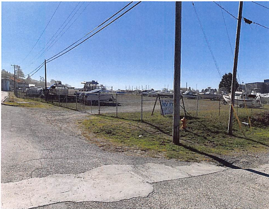
Resulting Area after Demo of "Green Building"
