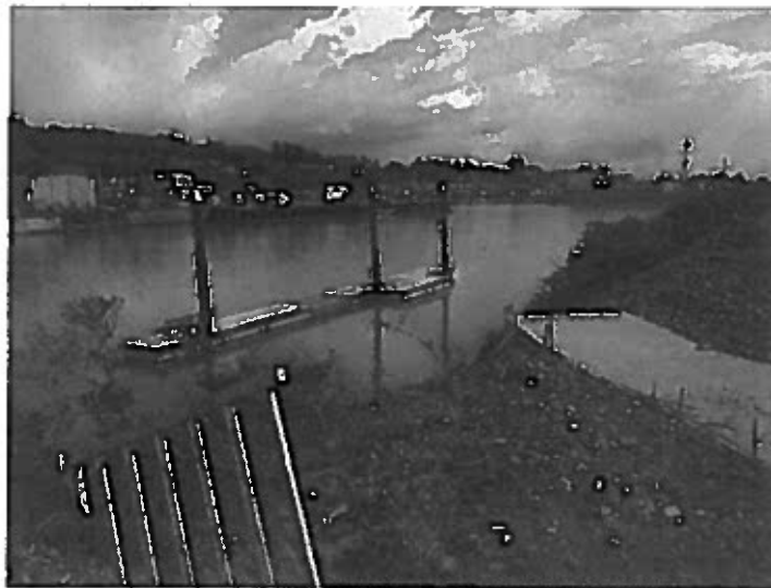
Photo 12 - Public fishing dock, abutment under construction
