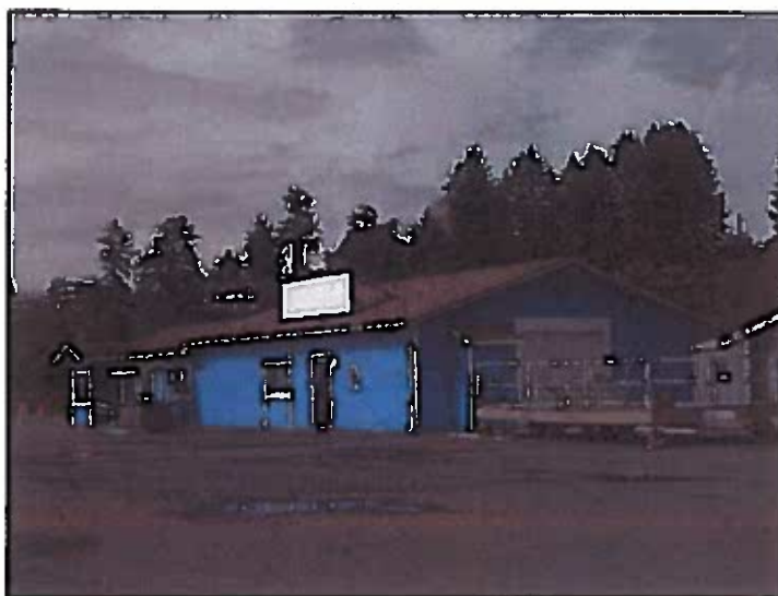
Photo 29 - Former cannery building
