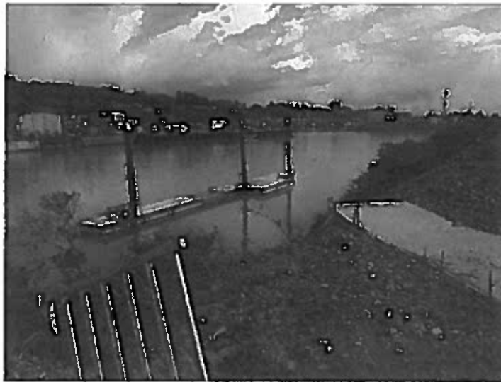
Photo 12 – Public fishing dock, abutment under construction
