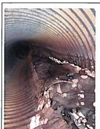
slide failure. Dirt and rock continue to flow out of the pipe. Condition of pipe is failing. Future plan for this area is filling in the barge area with Unknown amount of dirt and rock inside pipe. This culvert deposited large amount of dirt and rock from the 2015 Highway 101 sinkhole and dredging spoils and create new dock and land for Port use.
