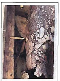
Manhole located in the boat launch parking lot has about 12 inches of dirt and rock. Dirt and rock increases in depth towards Fat Irish restaurant to about half the pipe.
