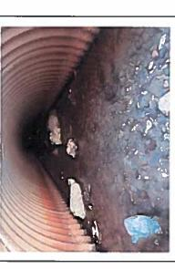
Culvert is half full of dirt and rock at the intake. 12 inches of dirt and rock in the pipe located at the manhole center of the parking lot. Large sediment removal. When culvert overflows, large amount of water flows through the retail parking lot and then impacts private property. amount of material deposited in Basin 1 that affected docks. Docks where removed and reconfigured to avoid more damage and future
