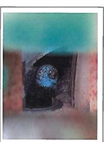
This culvert looks to be clear of dirt and rock. Sediment does flow from this culvert and into Basin 2. Drain intake at the edge of Lower Harbor Road may need to be upgraded.
