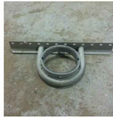
THE PHOTO ABOVE IS OF AN EXISTING HOOP AT THE PORT OF BROOKINGS HARBOR. THIS TYPE OF HOOP IS PREFERRED. THE BIDDER IS EXPECTED TO DISTINGUISH INSTALLATION OF DOCK-END HOOPS FROM THOSE INSTALLED ALONGSIDE DOCKS.
