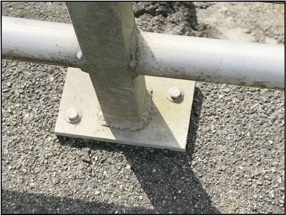
ACCESS PAD FENCE POST FASTENING
