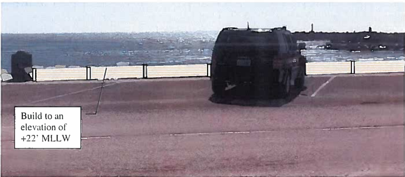
Vertical Repair Construction - Continuous
