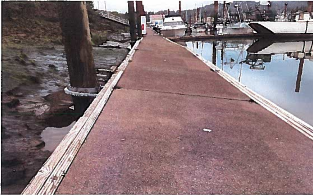
Docks hitting bottom between C & D, pictures taken May 8, 2016
