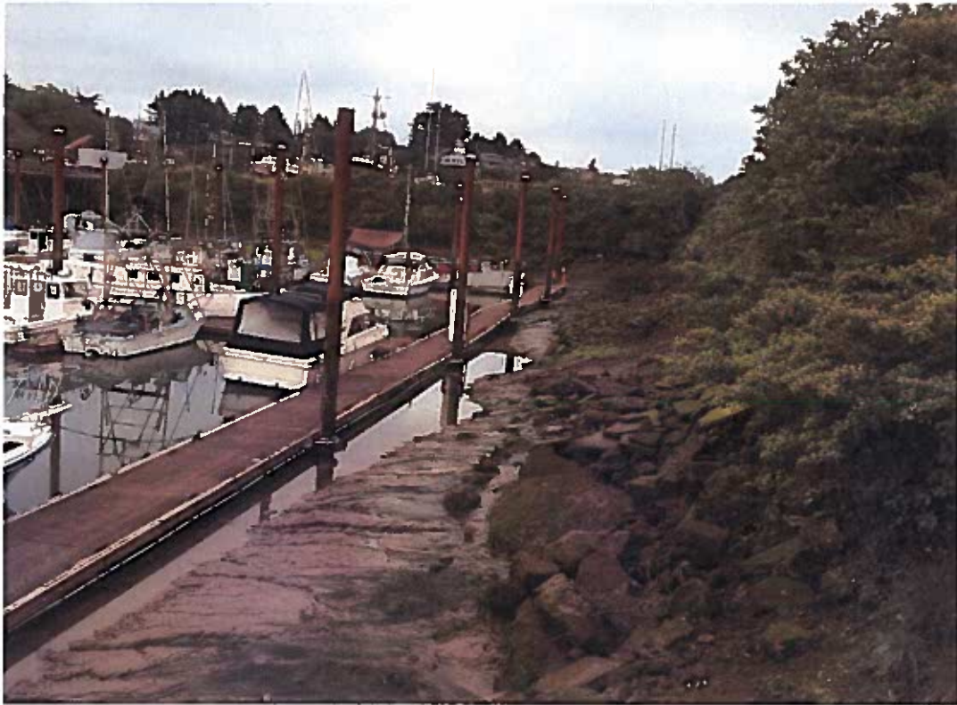
Ramp to H and I Docks hitting bottom at extreme low tide, picture taken on April 30, 2017.
