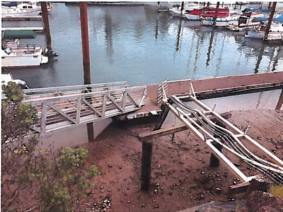
Ramp to H and I Docks hitting bottom at extreme low tide, picture taken on April 30, 2017.
