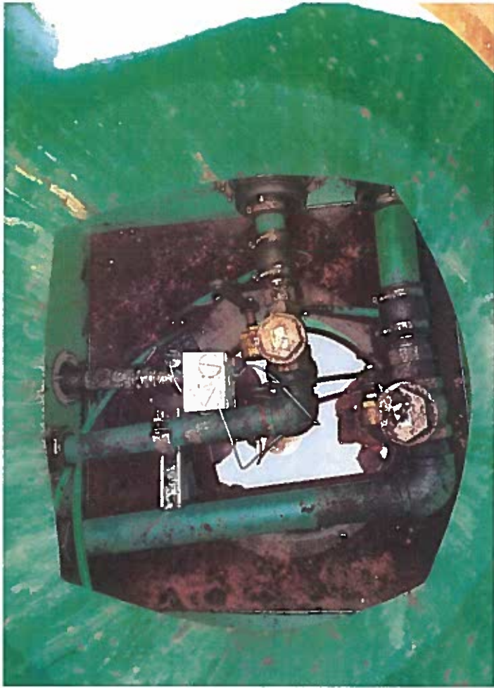
Breakaway valves installed, photo taken January 22, 2019
