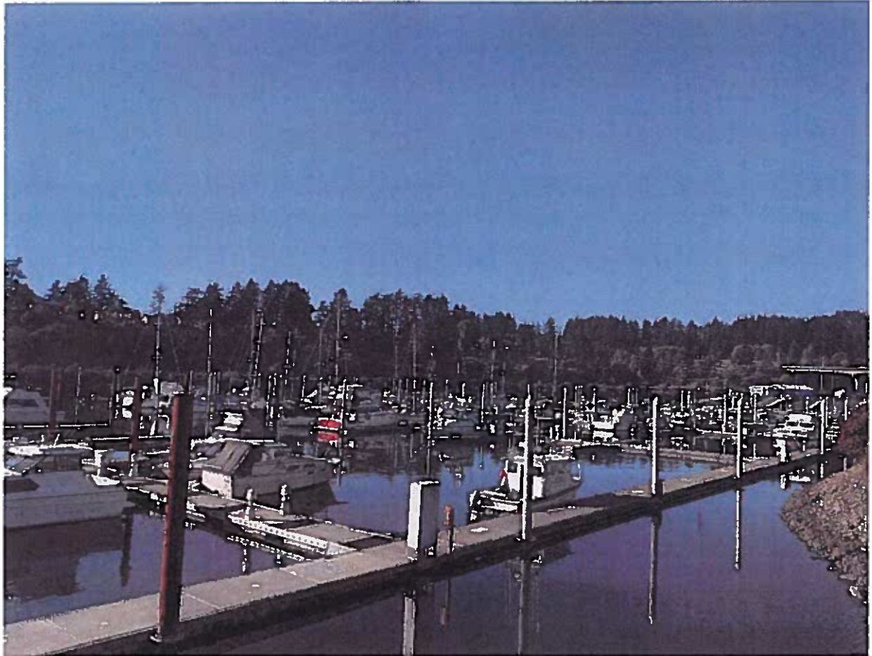
FEMA DR-4258 Basin 1 Piling Project completed April 2019
